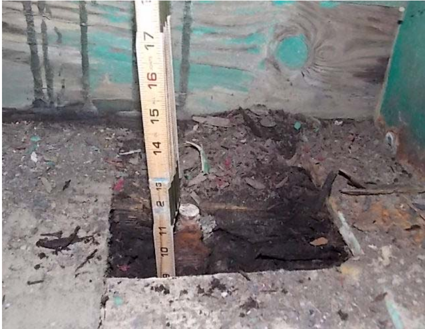
ABUTMENT # 1 CAP DECAYED OVER PILE "F"
