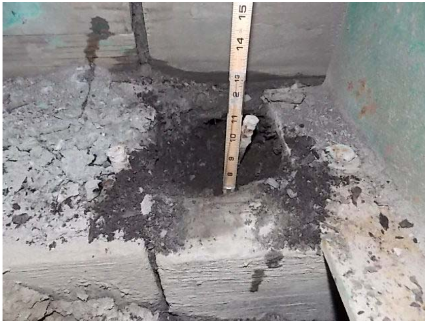
ABUTMENT # 2 TOP OF CAP DECAYED
