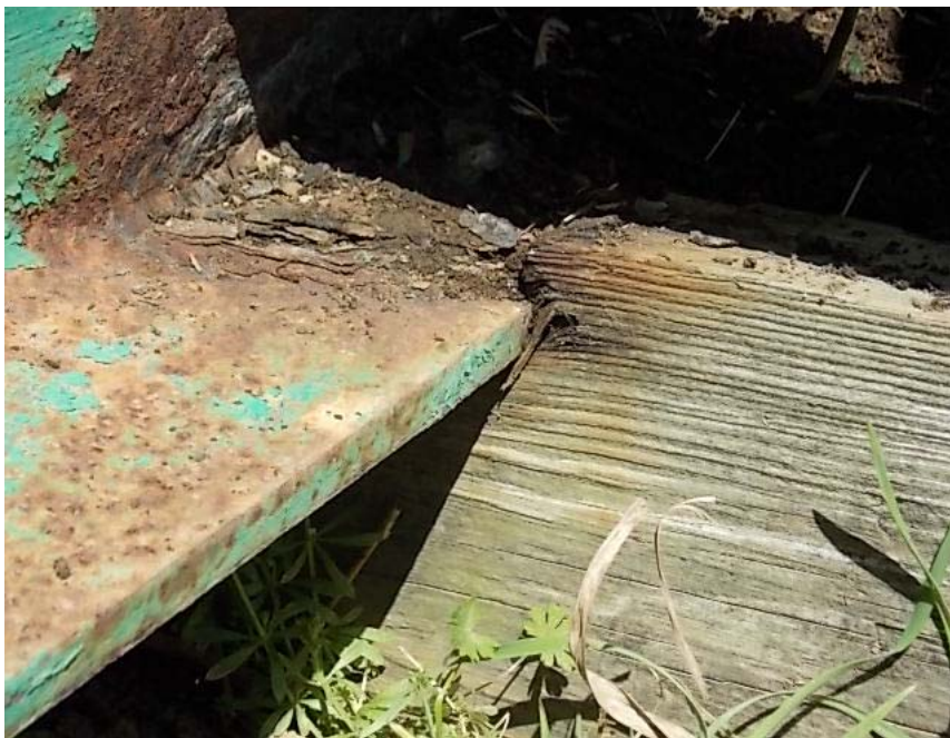
ABUTMENT # 2 RIGHT TOP OF CAP DECAYED
