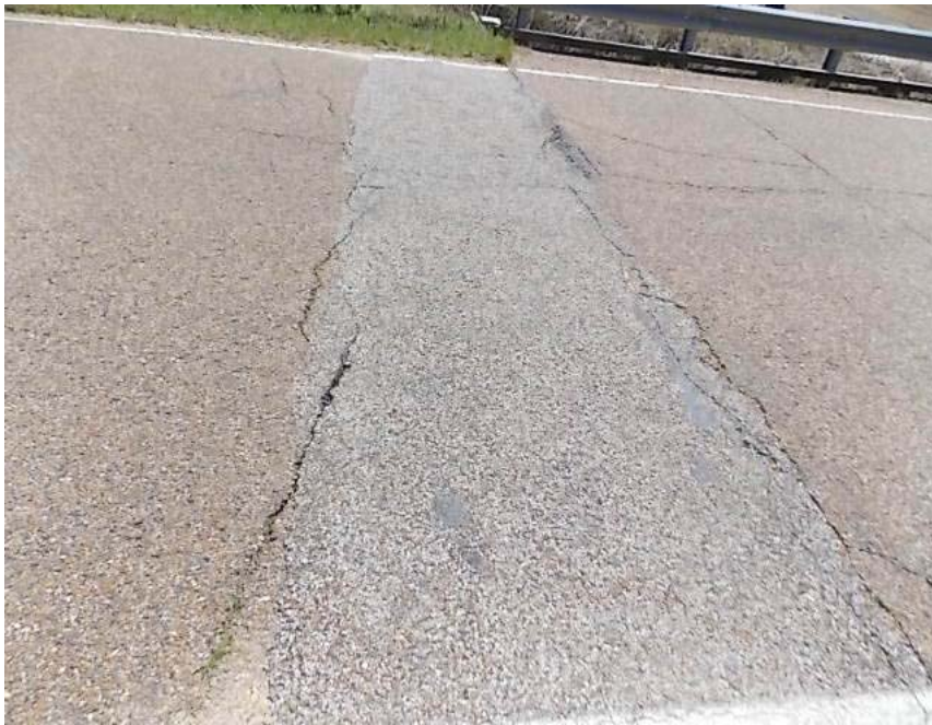
APPROACH # 2 A/C CRACKS
