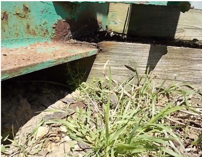
ABUTMENT # 2 RIGHT TOP OF CAP DECAYED
