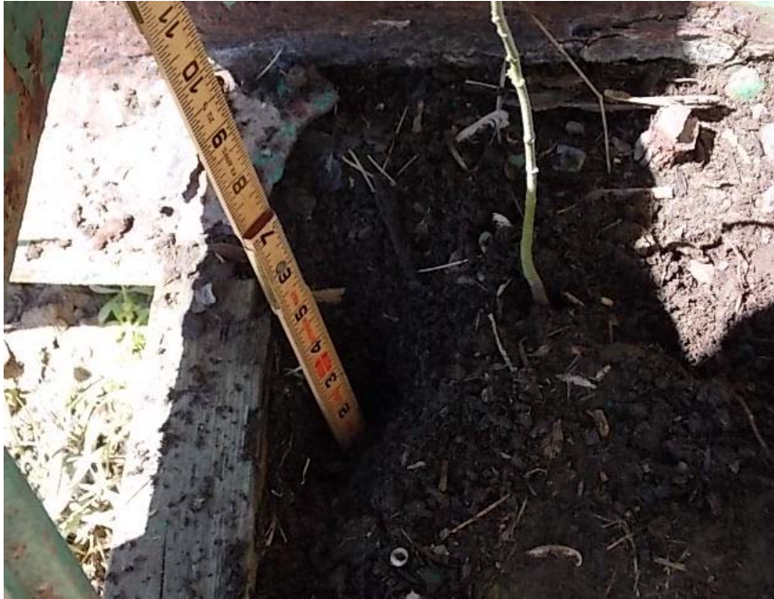
ABUTMENT # 2 RIGHT TOP OF CAP DECAYED
