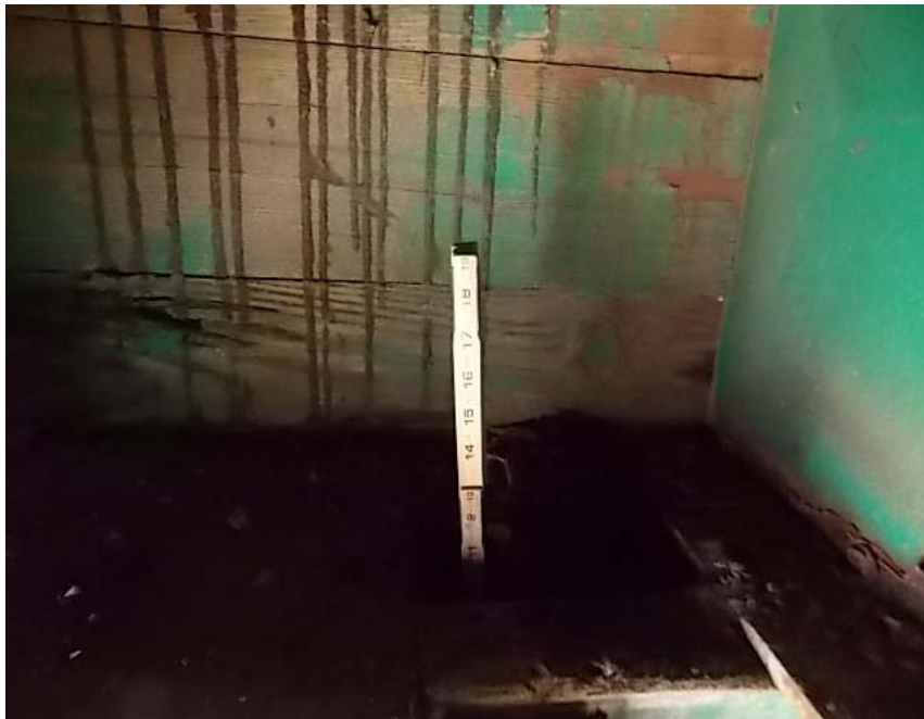
ABUTMENT # 1 CAP DECAYED OVER PILE "F"
