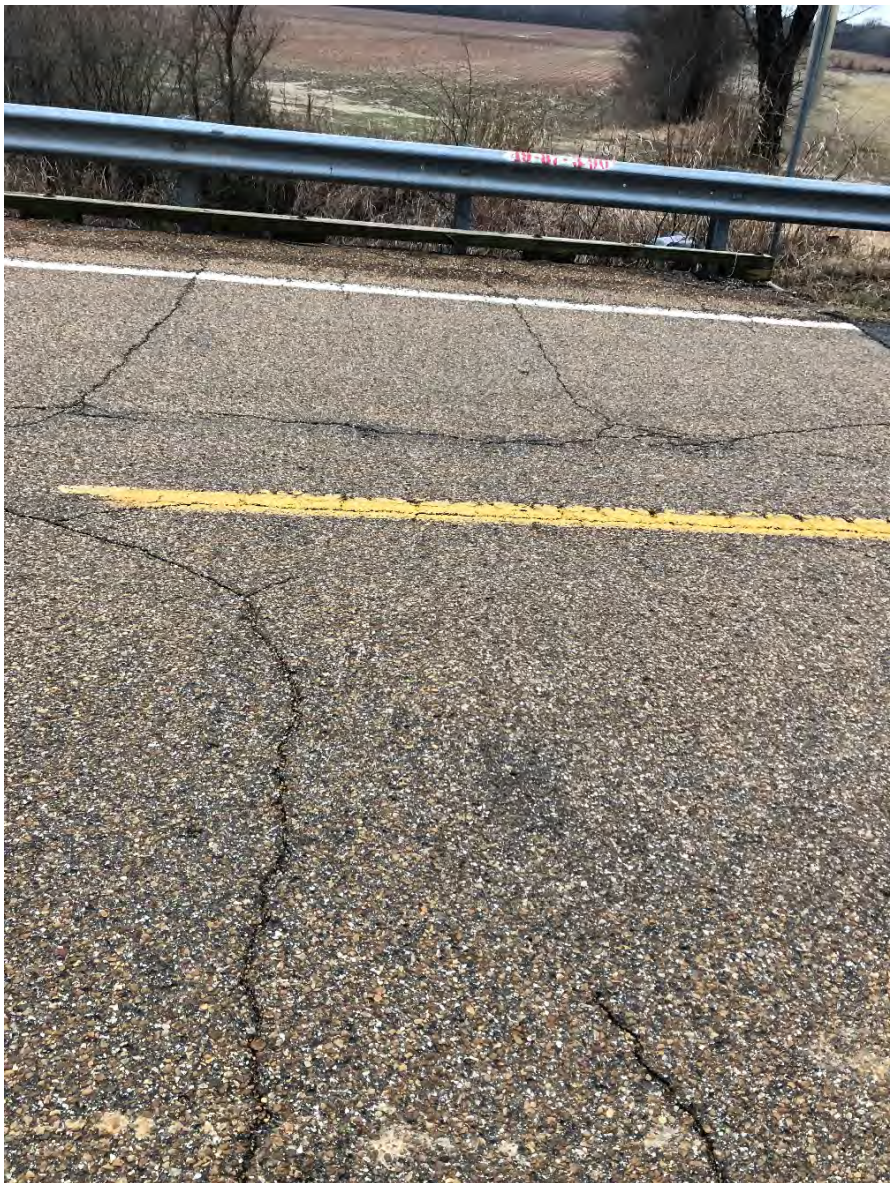
Severe Cracking on Bridge Surface
