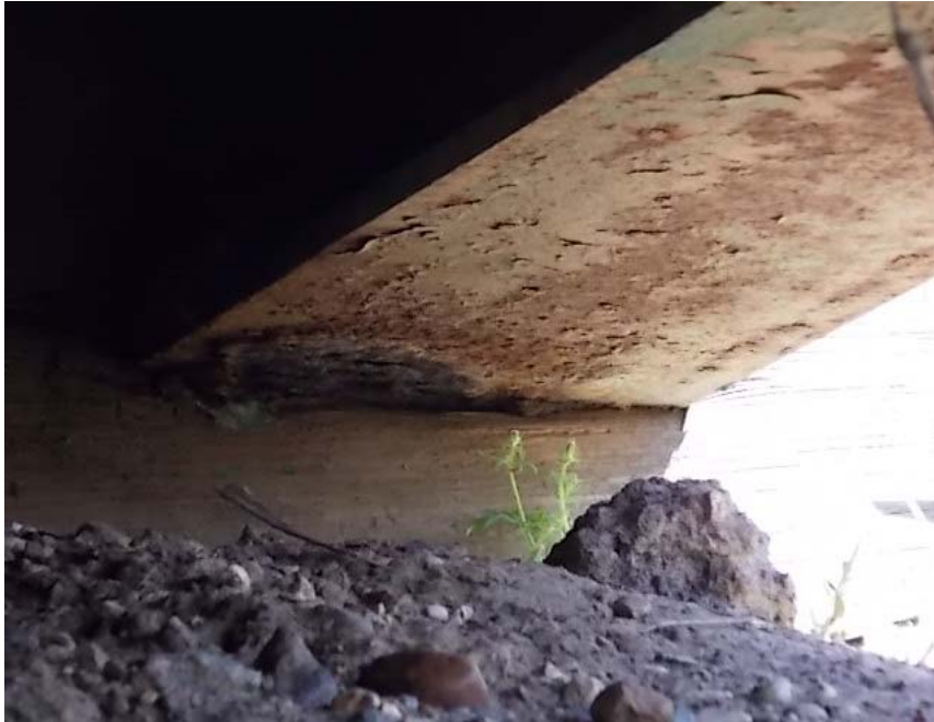
STEEL I BEAM "N" SETTLED TO ABUTMENT # 2 CAP
