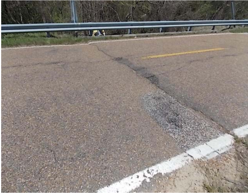
APPROACH # 1 A/C SETTLED & CRACKED
