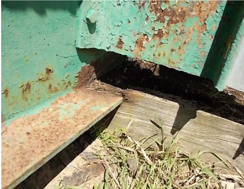
ABUTMENT # 2 RIGHT TOP OF CAP DECAYED
