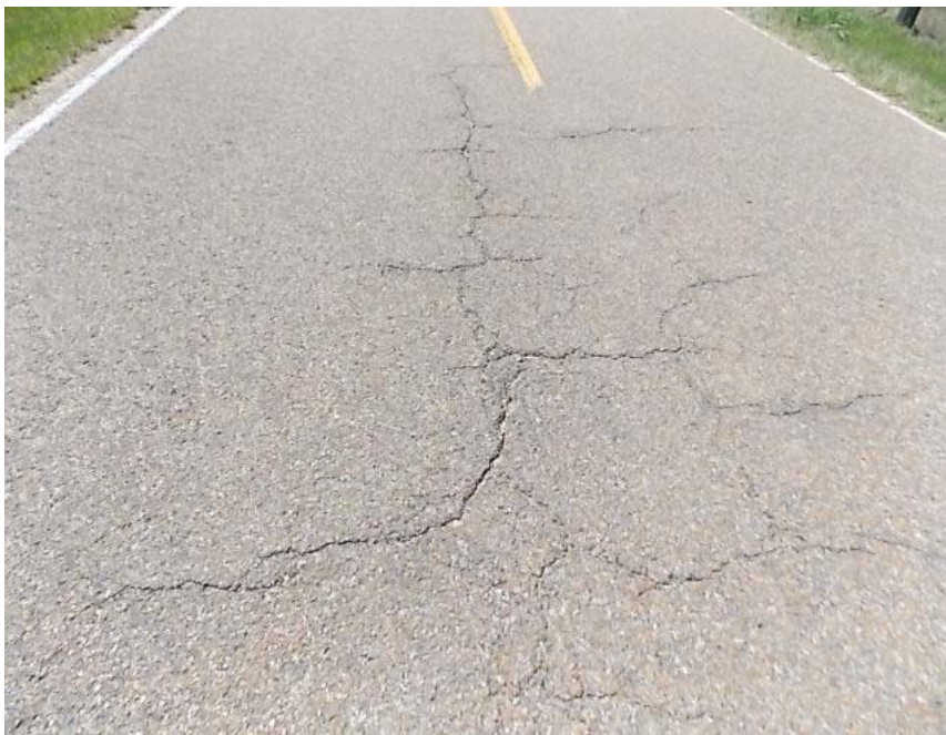
APPROACH # 2 A/C CRACKS
